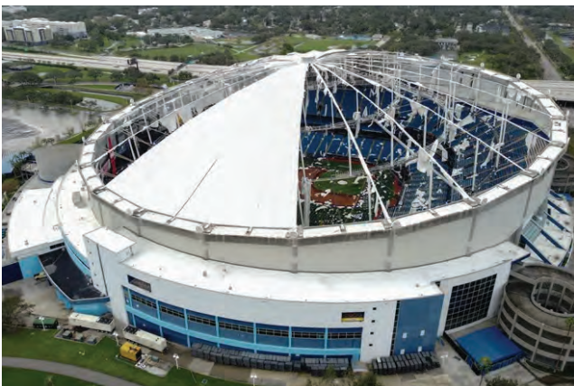
A drone image shows the dome of Tropicana Field which has been torn open due to Hurricane Milton in St. Petersburg, Fla., on October 10, 2024.
